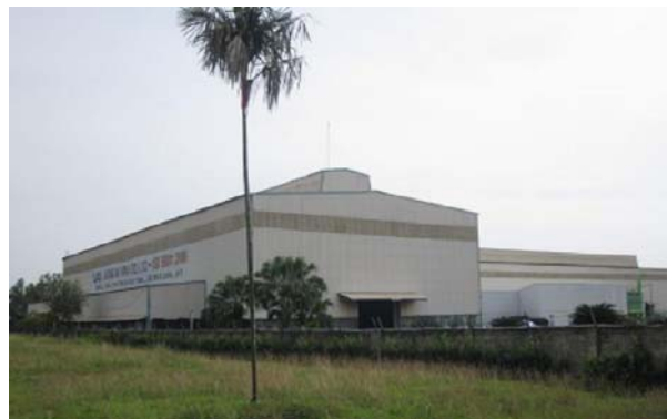
Jeong An Vina plant
