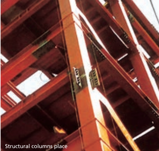
Structural columns place
