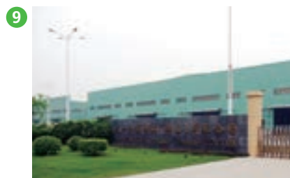
Maruichi Metal Product (Foshan) Co., Ltd. (MMP) Guangdong, China
