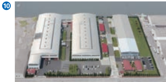
Shikoku Maruichi Steel Tube Ltd. Shikoku Plant
