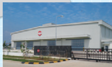
9 PT.Indonesia Steel Tube Works (ISTW) Cikarang Plant
