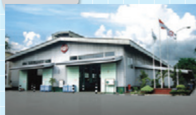
7 PT.Indonesia Steel Tube Works (ISTW) Jakarta Plant
