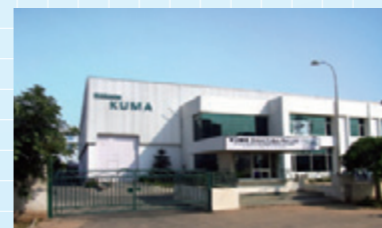
15 MARUICHI KUMA STEEL TUBE PRIVATE LIMITED (KUMA) MANESAR PLANT
