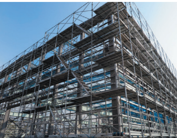
仮設用足場管 Scaffolding
