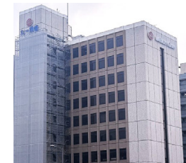
Former Headquarters (Kita-horie, Nishi-ku, Osaka City)
