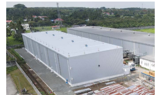
MPST's Second Plant Under Construction
